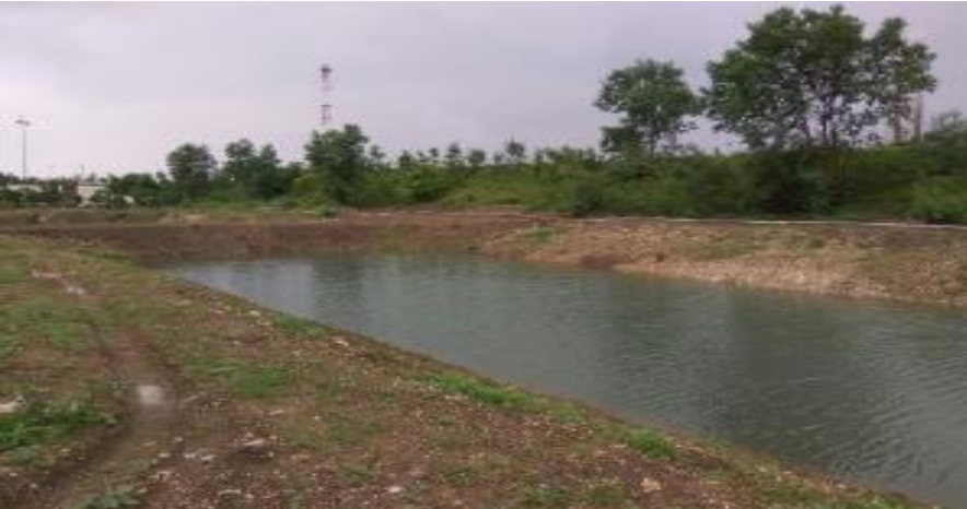
Rain Water Harvesting -54000 m3/annum recharge
